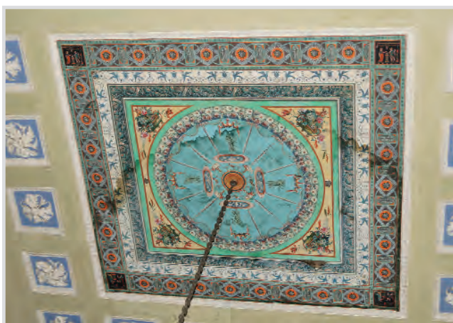
Fig 1 Italian Pavilion ceiling with decoupage appliques (©BaltStroy JSC)
