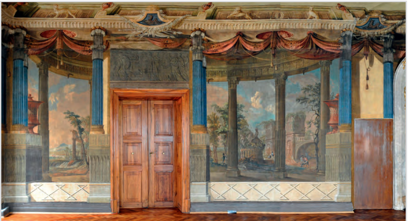
Fig 1: Total view of the west wall after conservation (© Krön)
